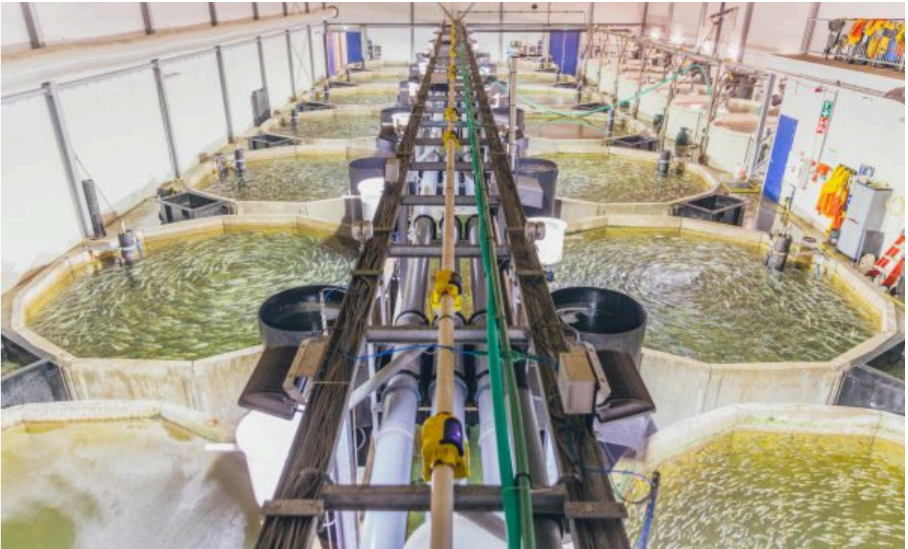
Figure 2.5: The structure of recirculating aquaculture system (RAS)
